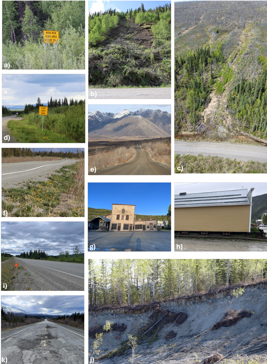
Figure 2. Compilation of field photographs documenting impacts of permafrost degradation in Yukon. Panel a) shows roadside sign marking a high-risk slide area outside Dawson City in Yukon. Panels b) and c) illustrate active-layer detachment slides adjacent to Alaska and Dempster Highways respectively. Panel d) indicates the termination of a slide-affected road segment. Panels e) & f) show road deterioration of the Dempster and Haines Highways respectively. Panels g) & h) show buildings in Dawson City, affected by permafrost degradation. Panels i) & k) document cracking and subsidence. Panel j) presents an exposed retrogressive thaw slump scarp. Photos: Eirini Makopoulou.
